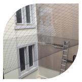
NETTING. This is the most permanent and economical way to prevent access for any species of bird. A stainless steel wire with a high quality netting is installed around an area, providing a very secure solution and long term results.
